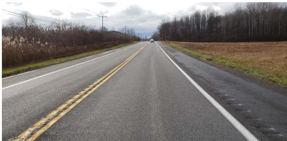
Figure 14. Two-Lane Highway with Centerline and Shoulder Rumble Strips
