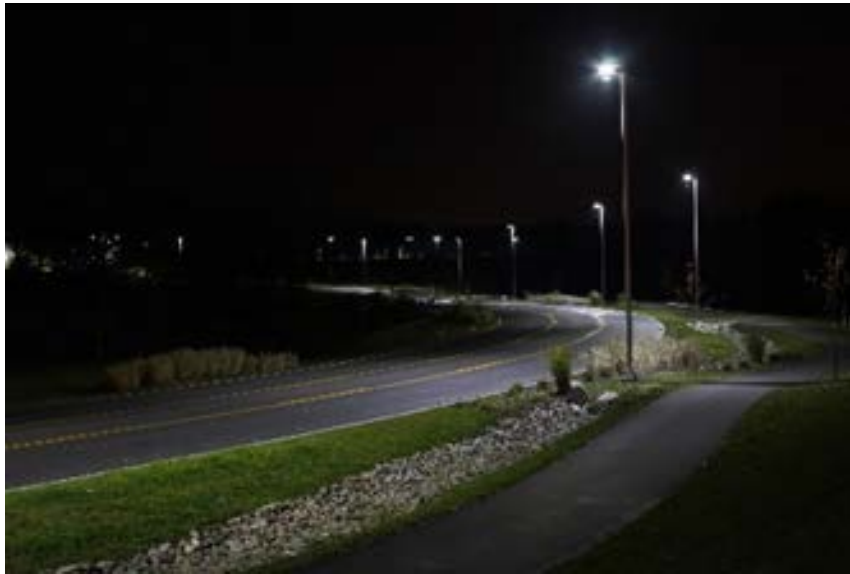
Figure 15. Horizontal Curve Lighting
