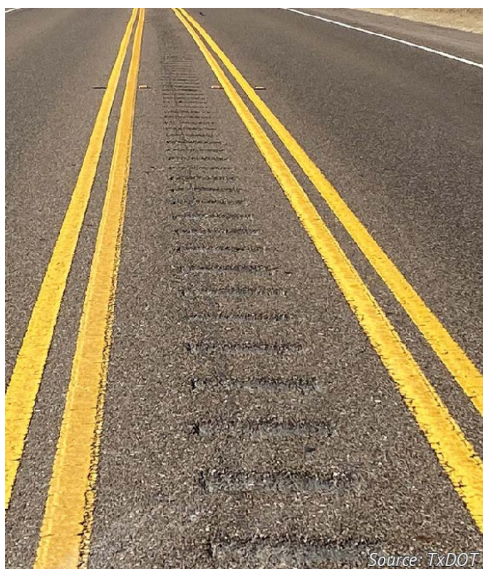
Figure 18. Centerline Buffer.
