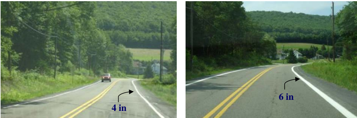
Figure 12. 4-Inch (Left) and 6-Inch (Right) Edge Lines in Rural Two-Lane Roads
