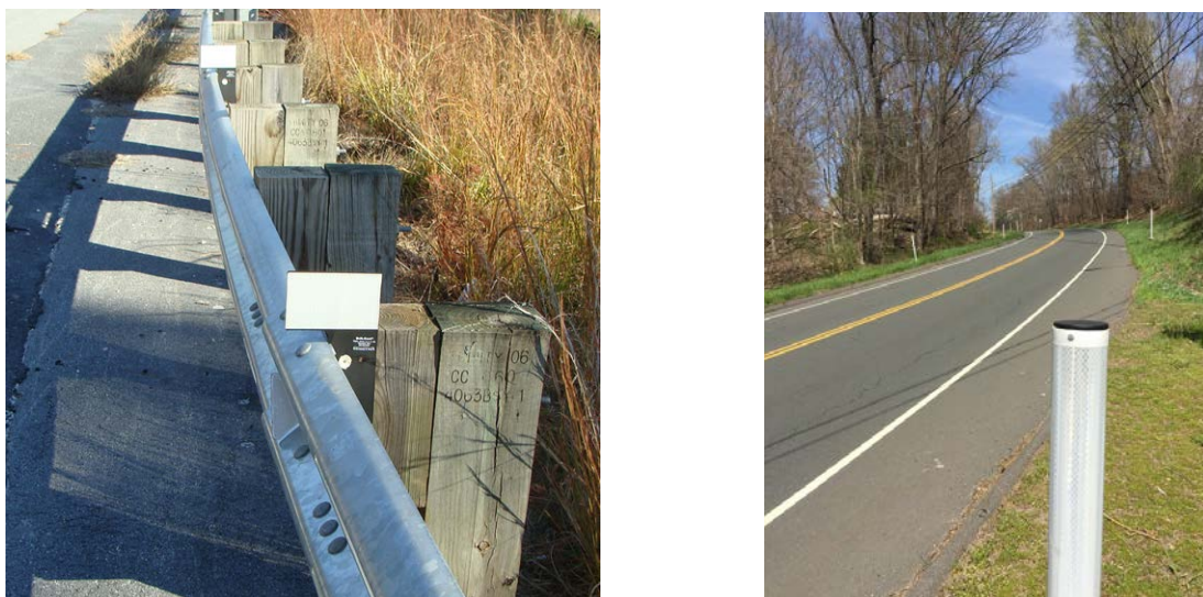
Figure 13. Barrier Mounted and Post Mounted Delineators
