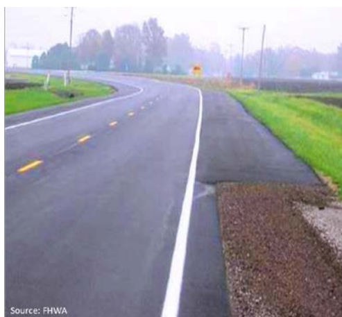
Figure 16. Horizontal Curve with Widened Outside Shoulder
