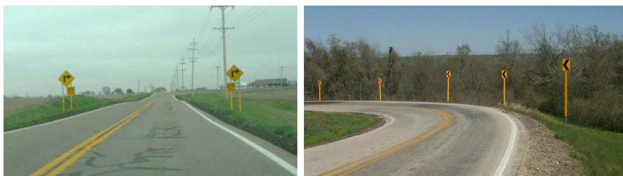
Figure 10. Horizontal Curves with Signs and Chevrons
