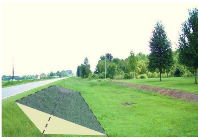
Figure 21. Traversable Slope
