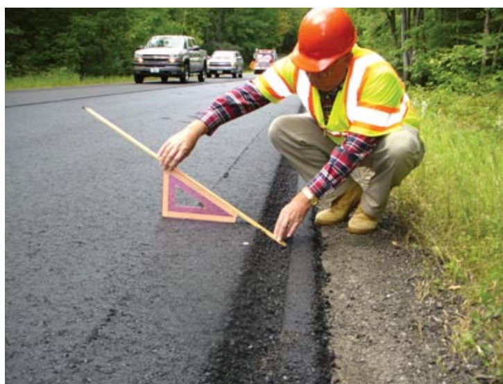
Figure 17. Safety Edge
