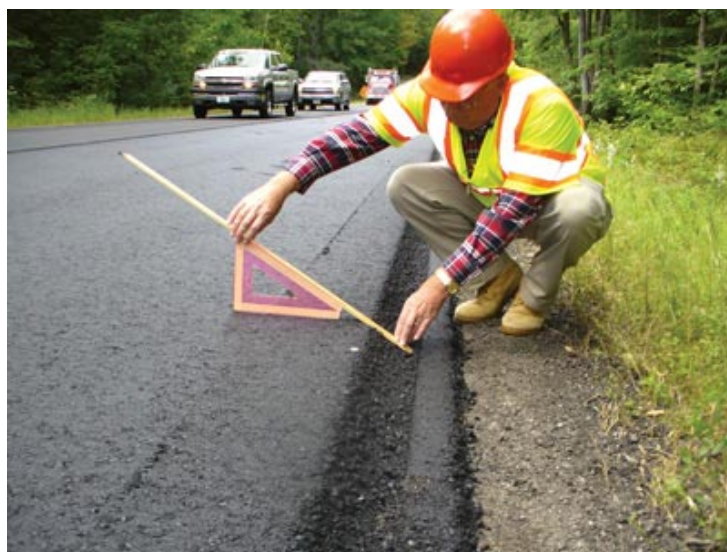
Figure 17. Safety Edge
